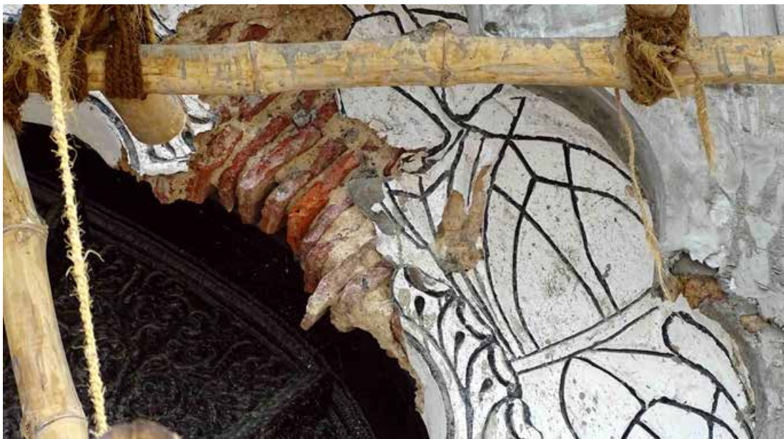
Image 9: A cusped arch made of Lakhauri bricks at the Chota Imambara, https://anotherglobaleater.files.wordpress.com/2015/08/ci-lakhauriarch.jpg
