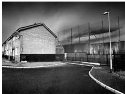
Fig. 13 This photograph shows the project developed by Seán Mackel recreating the street destroyed by the bombing in the two most turbulent of the Troubles, increasing technical standards and providing decent housing for families that lost all their houses as a result of the conflict. Image copyright Ciaran Mackel's archive
