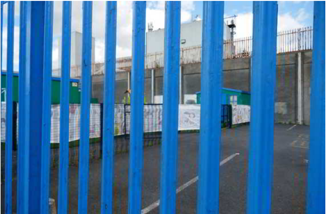
Fig. 6 In this image taken also at the bottom of the Falls, there are four defensive devices in a children playground area, 1- Palisade security fencing in blue 2- A black metal fence acting as a defensive barrier outside the children's' playground area 3- Brick wall in grey concrete 4- Metal fence on top of the wall. Image copyright Alona Martínez Pérez
