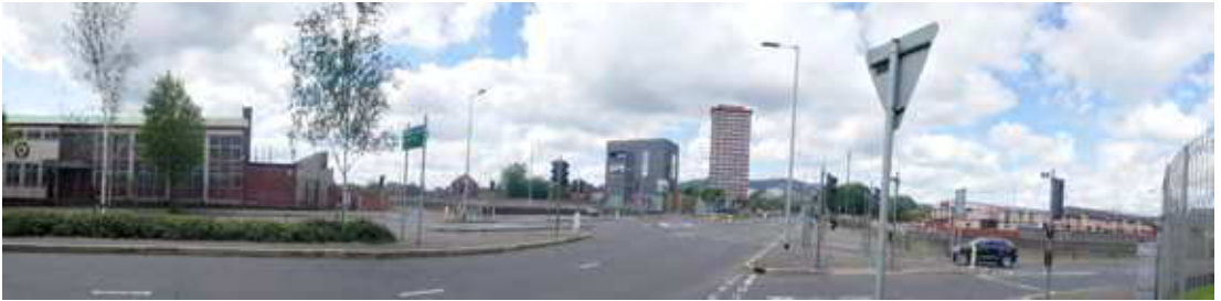
Fig. 9 In this image the street landscape is fractured by the Westlink motorway, a car-oriented environment full of car signs that does not welcome pedestrians. The building Raidió Fáilte designed by architect Ciaran Mackel provides a positive landmark and intervention in such a complex post-conflict, post 1960's urban landscape with the Divis Tower to the right Image copyright Alona Martinez Perez
