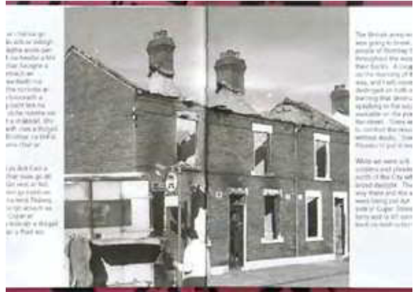
Fig. 12 Image showing the destruction of Bombay Street after the houses were burnt to the ground Image copyright Ciaran Mackel's archive
